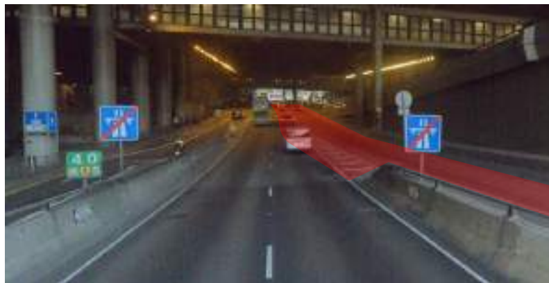
觀塘繞道東行下行斜道 Kwun Tong Bypass Eastbound Downramp
